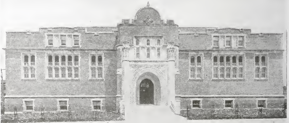
HOMEWOOD BRANCH, CARNEGIE LIBRARY, PITTSBURGH, PA. Alden & Harlow, Architects, Pittsburgh, Pa.
